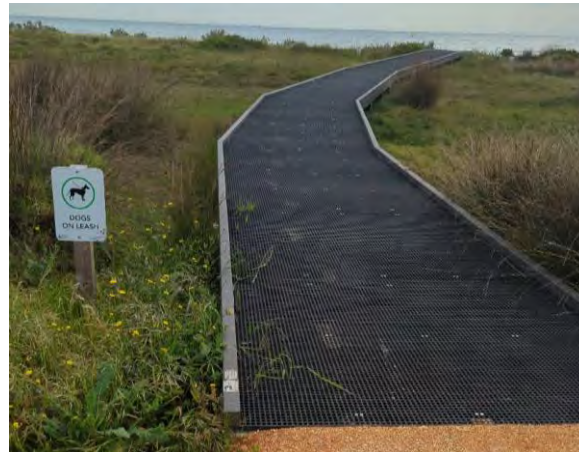
Figure 6-5 All Abilities access north of Indented Head near Coach Road
